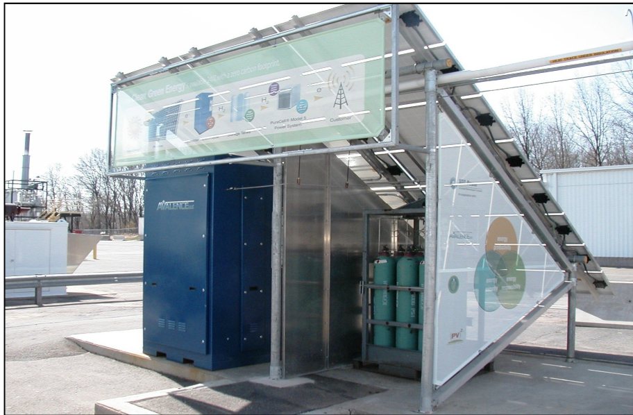
Solar Powered Back-Up Power System at UTC Power, Windsor, CT
