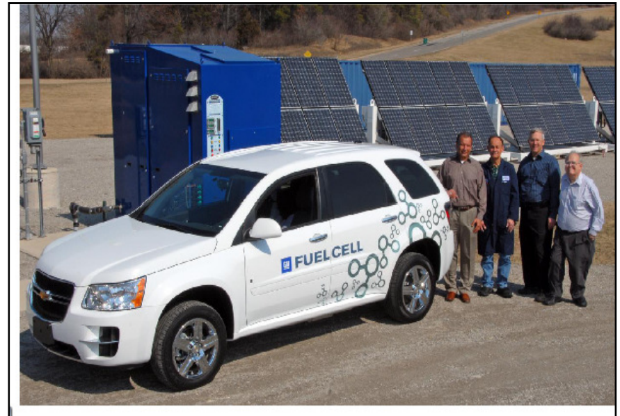
Complete Solar Powered Hydrogen Fueling Station at General Motors, Milford, MI
