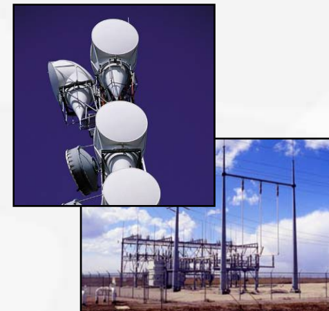
Telecommunications Critical Backup/ Emergency Power
