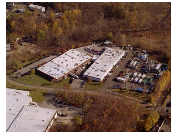
Danbury, CT - Headquarters, R&D, Stack Conditioning
