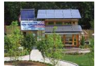
Renewable Energy Storage
